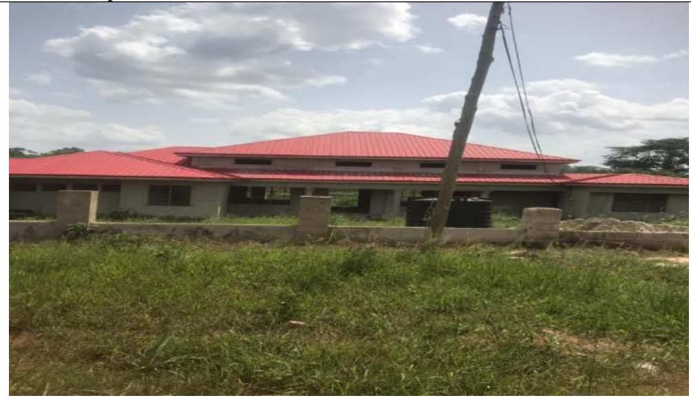
District Court Complex
