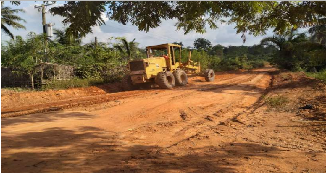
Reshaping of 16km road from Kwapong Junction to Agyarekrom
